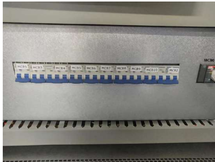
Figure 9-1: Internal circuit breakers of BCP (For reference only)
