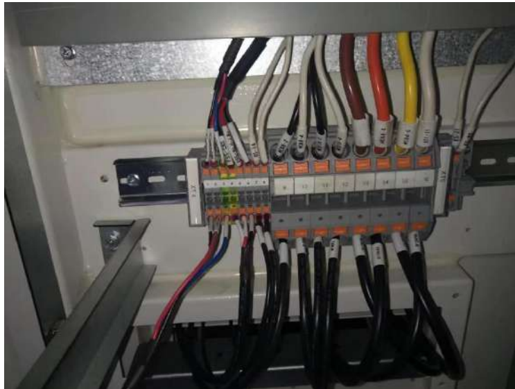
Figure 8-13: The XT4 terminal block in the BCP (For reference only)
