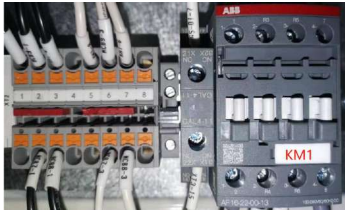
Figure 8-24: UPS maintenance bypass
