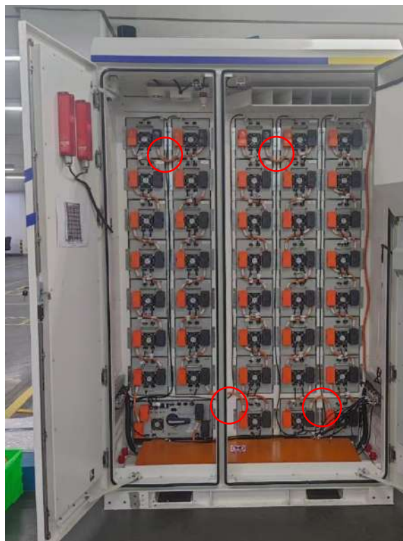
Figure 6-1: Cables need to be disconnected(for reference only)
