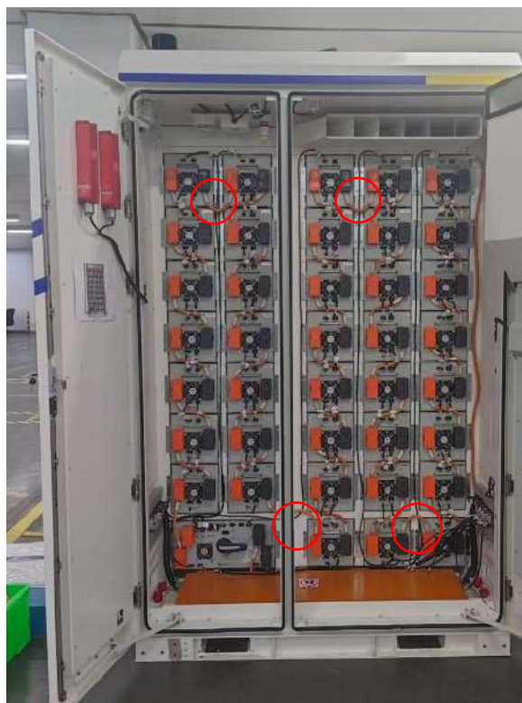
Figure 8-20: Location of the removed jumper
